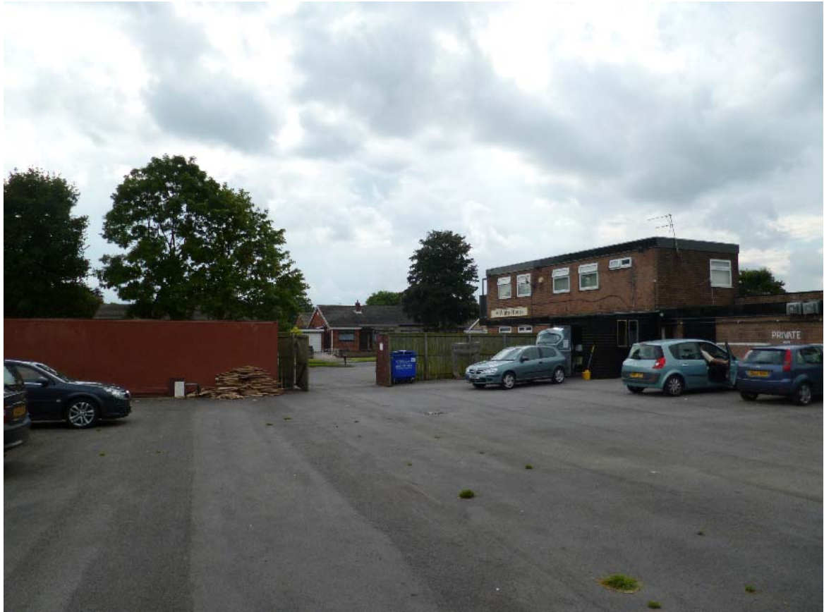
View of extension and container from yard area
